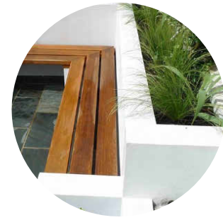
REN-01 Blockwork Rendered Paint Finish - White
